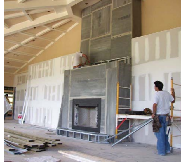
Veranda, under construction
