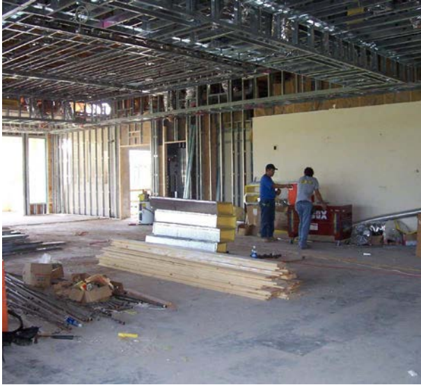
Formal dining room, under construction
